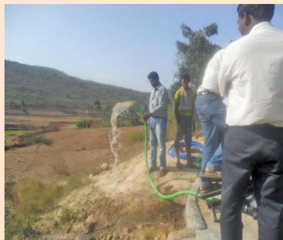
During the trial, the pump lifted water up to 23 ft.
