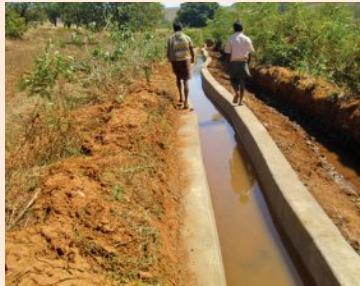
Masonry canal
