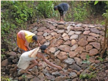
Loose Boulder Structure
