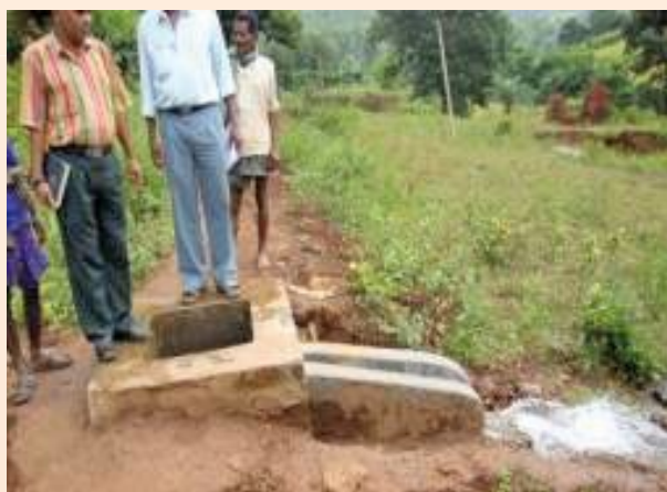
Outlet of a Diversion based irrigation project
