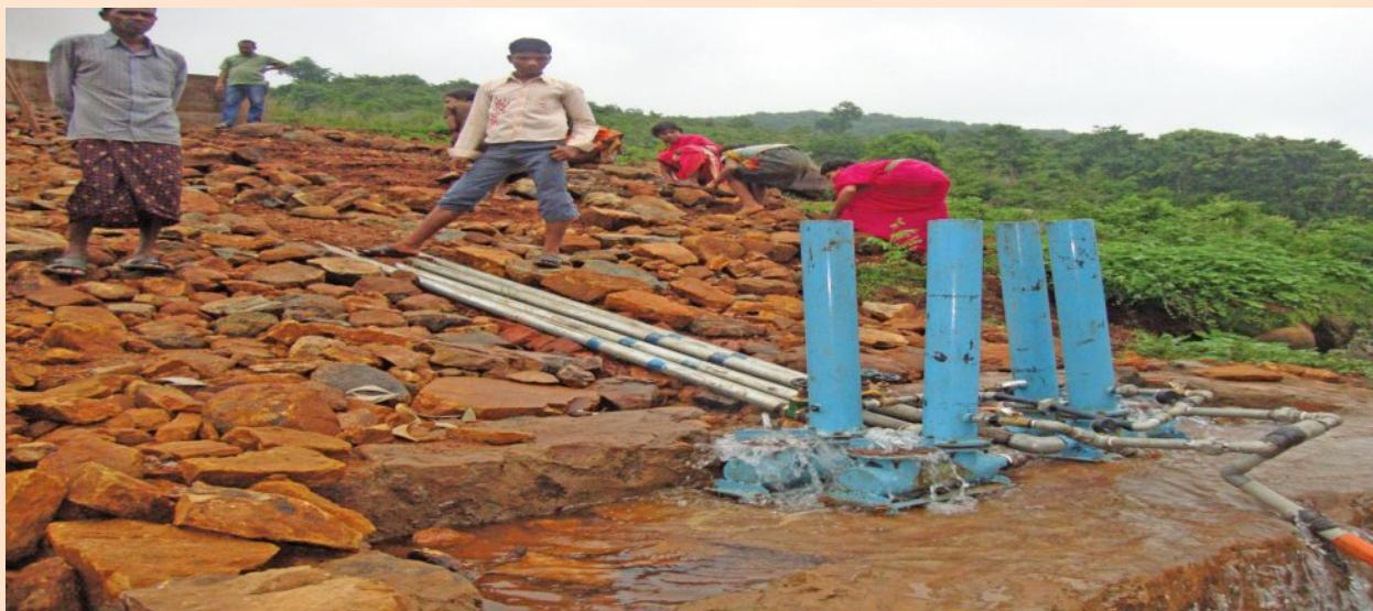
Operation of 4 nos. of hydrams in series
