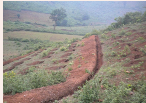
Contour and Staggered Trench
