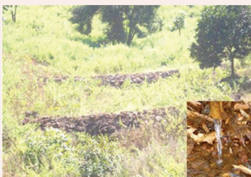
Series of Gully Control structures created across streams. Evidence of seasonal streams becoming perennial (corner photo)
