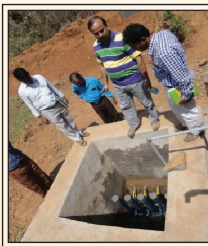
Hydram project for upland irrigation and domestic use
