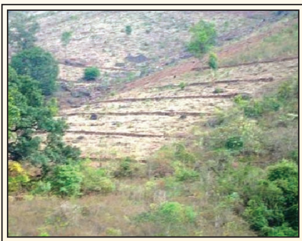
Stone bunds in series in shifting cultivation patches
